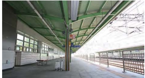
세마역 전기공사 Platform Electrical Work of Sema Train Station
