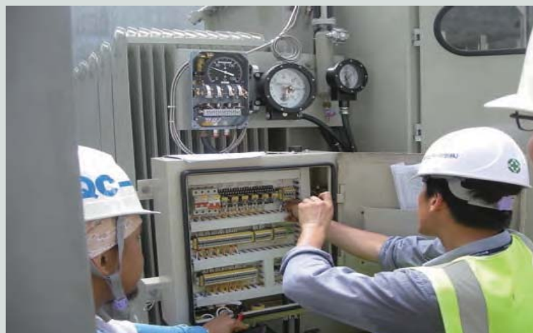
단말처리작업 Cable Termination Work
