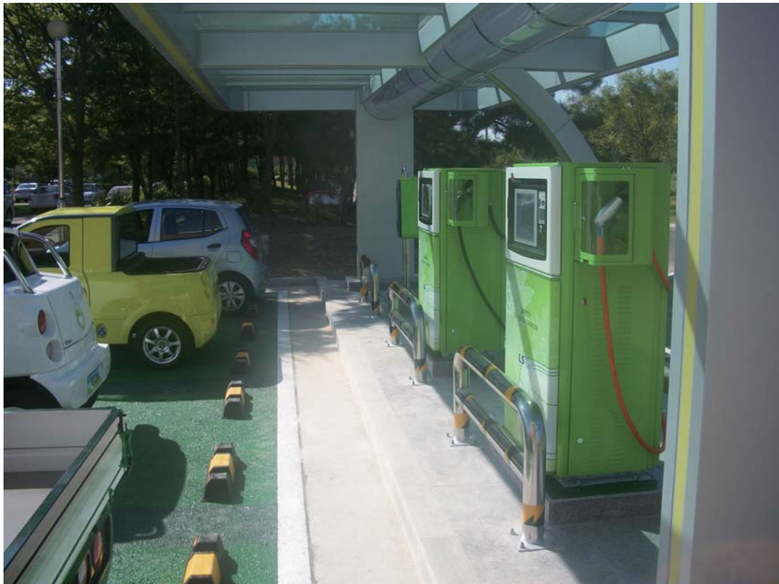
전기자동차 충전소 설치 공사 Installation Work of Electric Vehicle Charging Station
