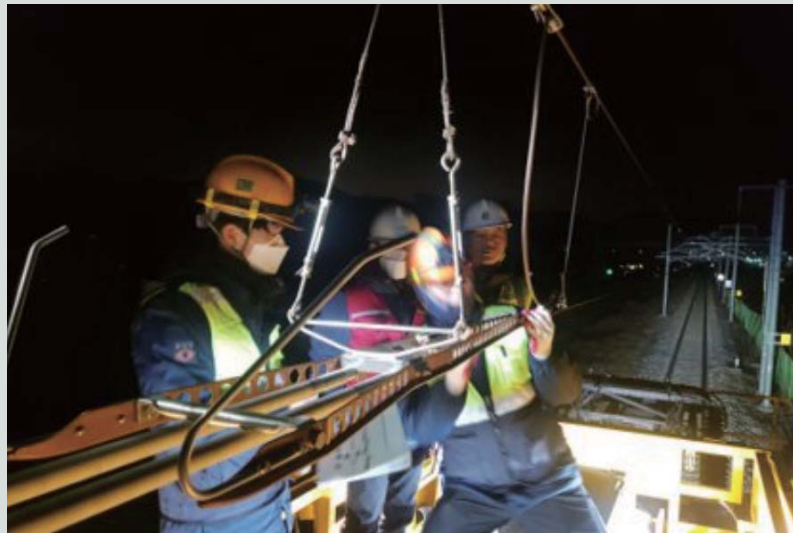
철도전차선공사 Electric Train Track Construction
